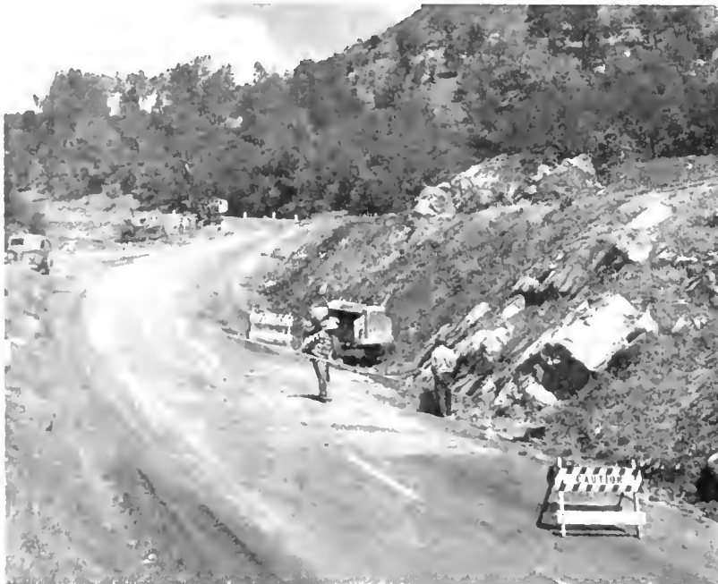
LEFT—Drilling for blasting on portions to be realigned. RIGHT—Portion of existing road to be widened and resurfaced. No change in alignment to be made.
